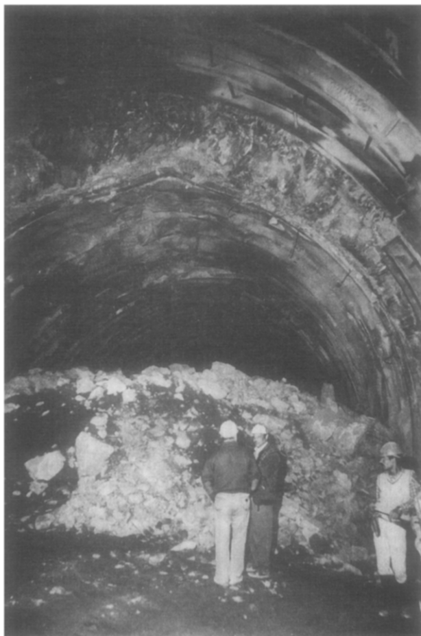
Fig. 16. large displacements in the top heading of the headrace tunnel of the nathpa Jhakri hydroelectric project in India.
