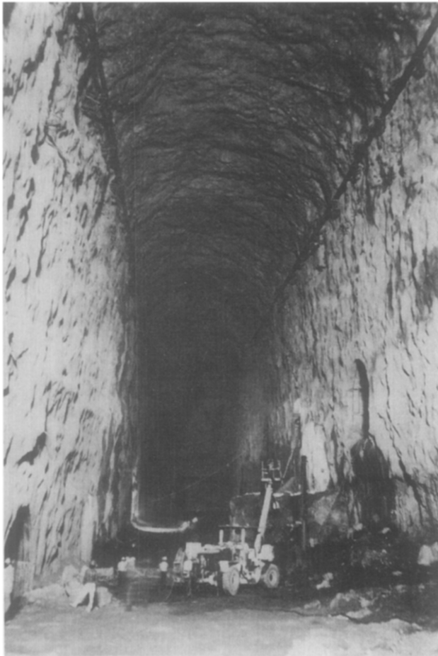
Fig. 14. Partially completed 20 m span, 42.5 m high underground powerhouse cavern of the Nathpa Jhakri Hydroelectric project in Himachal Pradesh in India. The cavern is approximately 300 m below the surface.
