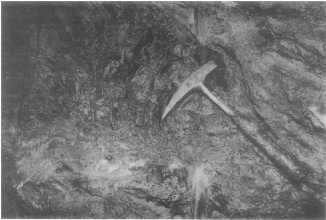
Fig. 20. Appearance of the very poor quality Athenian schist at the face of the side heading illustrated in Fig. 19.
